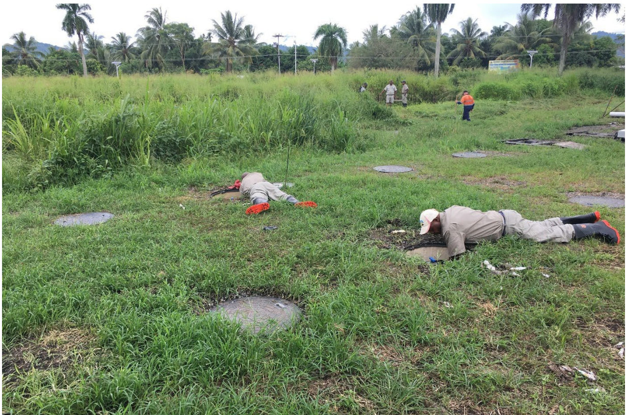
Figure 31 – Onsite personnel that have been trained by True Water technicians inspecting the chambers of the STP modules.
