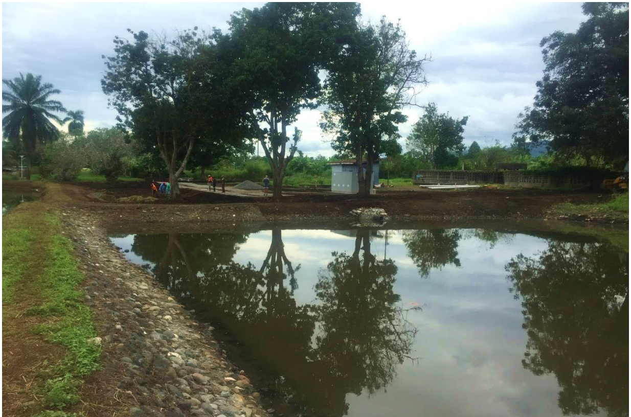
Figure 26 – The STP treatment chain ends in this storage pond.
