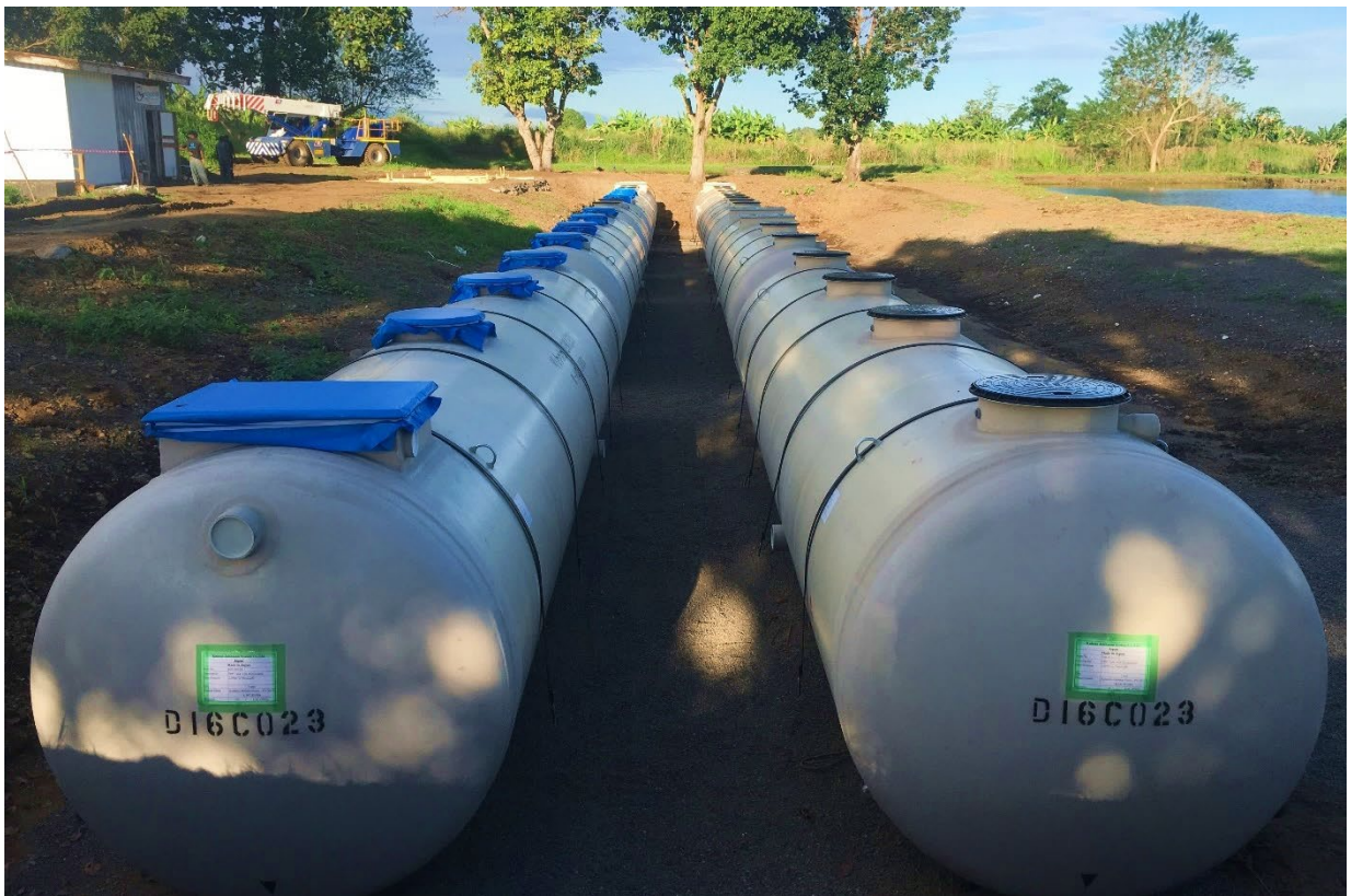
Figure 14 – STP modules in position and level prior to interconnection and anchoring.
