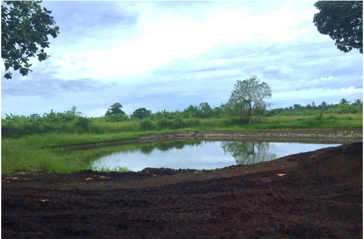
Figure 25 – The existing holding ponds for the treated wastewater were in good condition.
