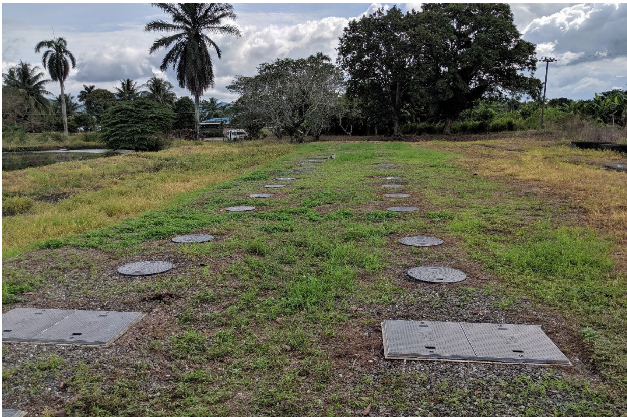
Figure 35 – The Igam Barracks sewage treatment plant five years after delivery.
