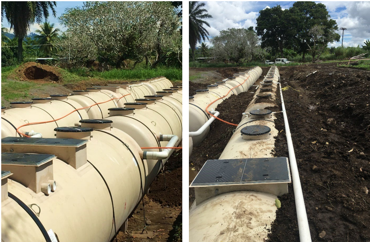
Figure 16 – STP modules connected in a treatment chain and partially backfilled.
