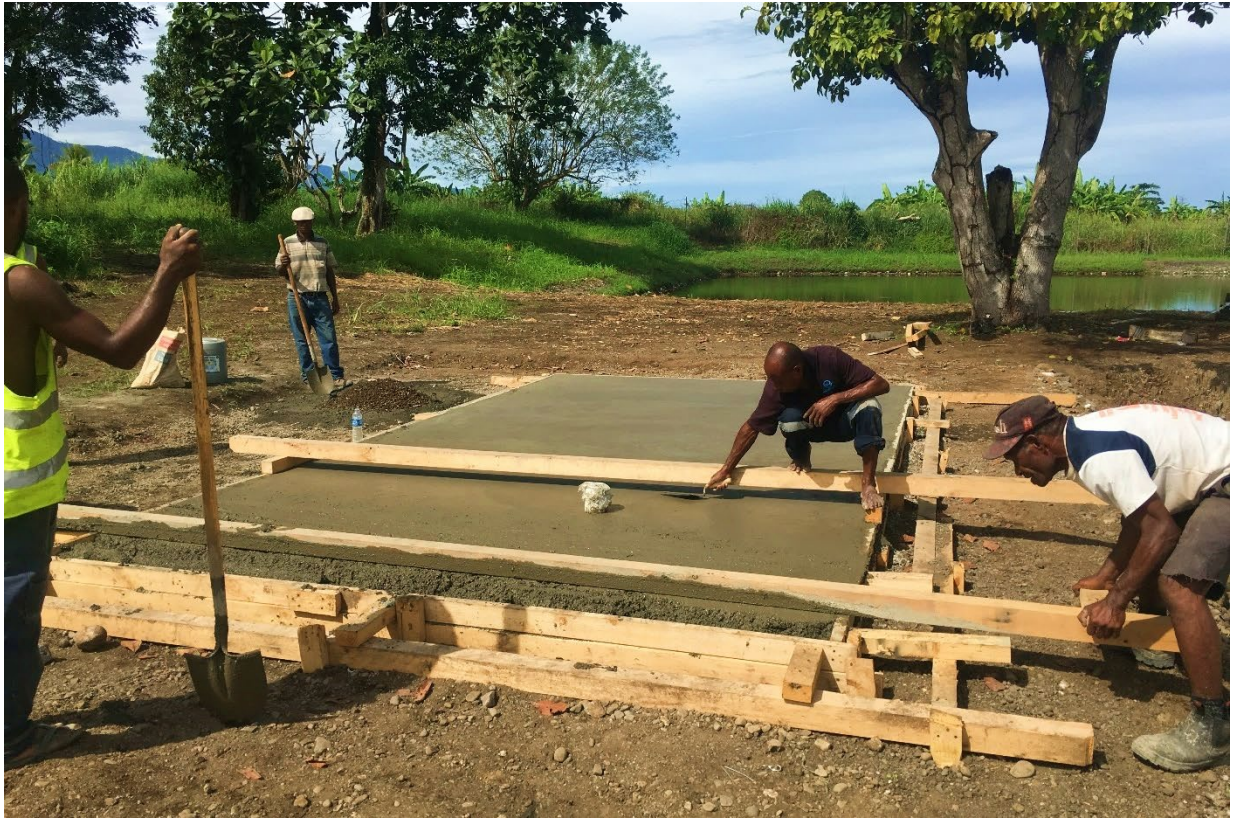
Figure 17 - Concrete slab preparation for Control Room.
