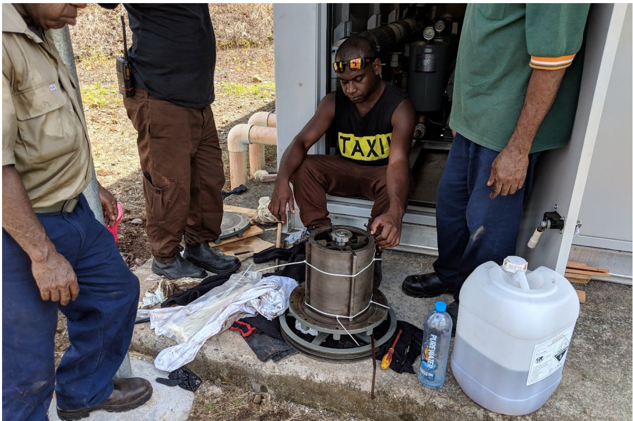
Figure 33 – Onsite personnel completing air pump maintenance training.
