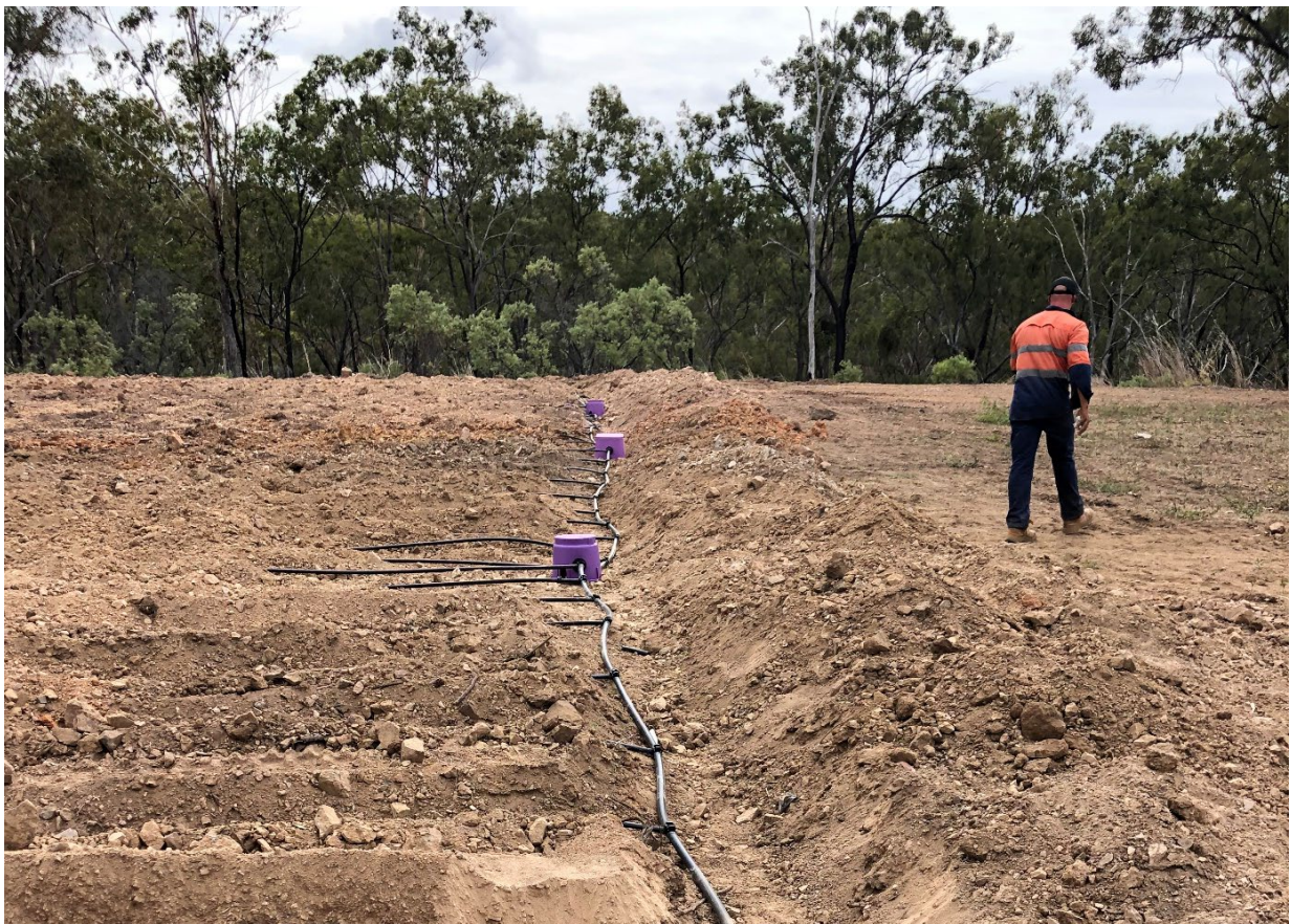
Figure 24 – Installation of sub-surface drip irrigation
