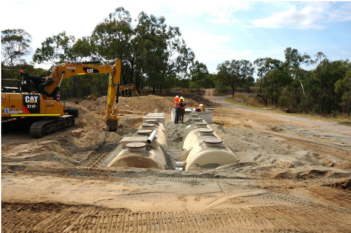
Figure 17 – Kubota STP with partial backfill
