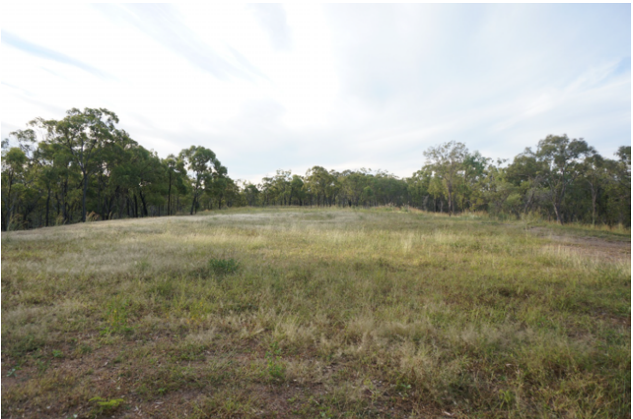
Figure 26 – Sub-surface irrigation area eight weeks post installation
