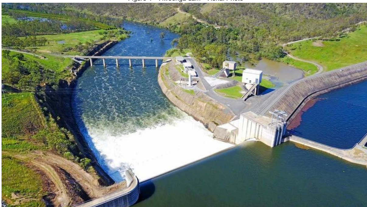
Figure 4 – Awoonga dam – Aerial Photo
