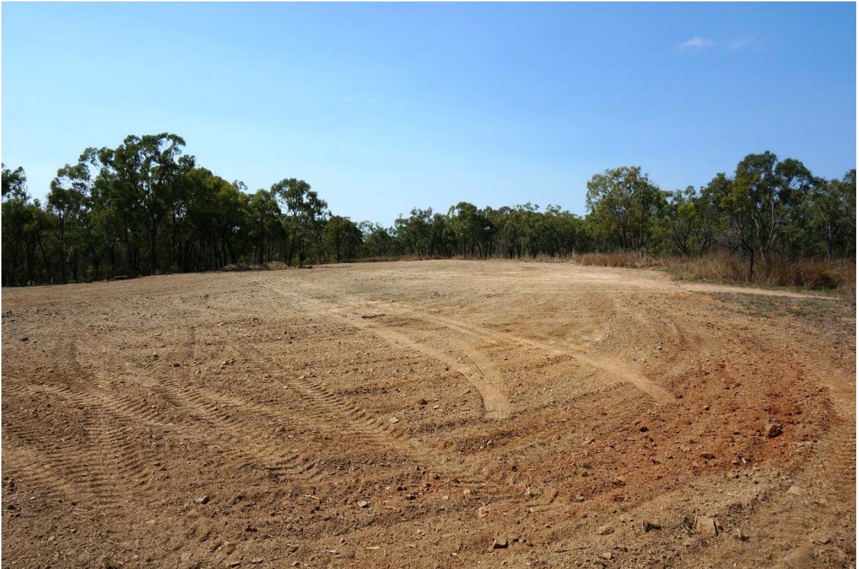
Figure 25 – Completion of Sub-surface irrigation field
