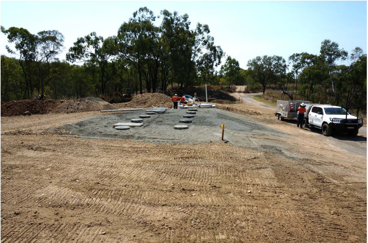
Figure 18 – Kubota STP with complete backfill
