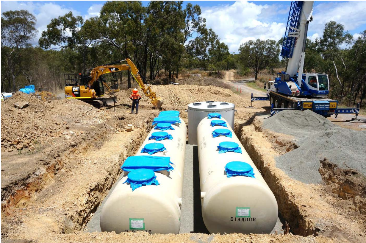
Figure 16 – Kubota STP prior to backfill
