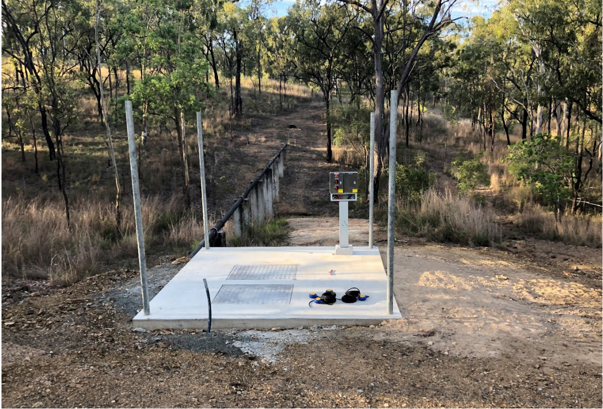
Figure 20 – Delivery Sewage Pump Well finished slab, prior to fencing
