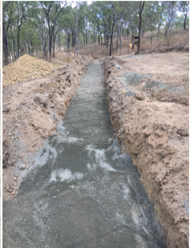
Figure 22 – Services trenching with select material cover
