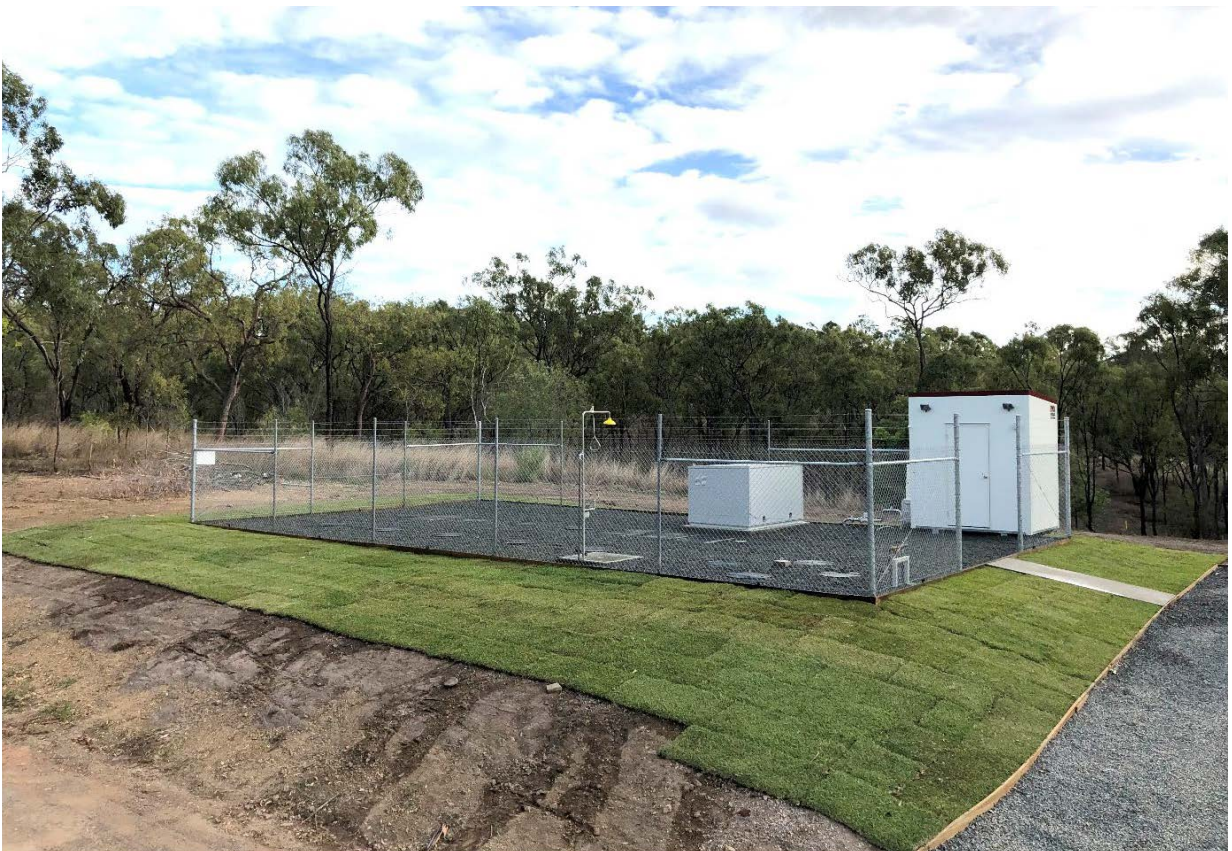
Figure 19 – STP compound with finishing
