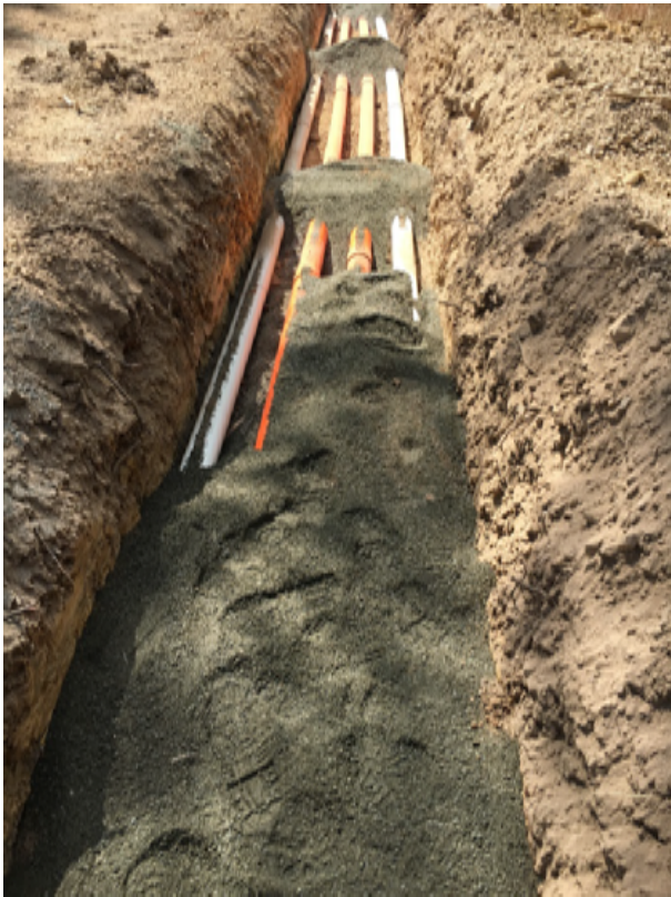
Figure 21 – Servicing trenching with partial cover
