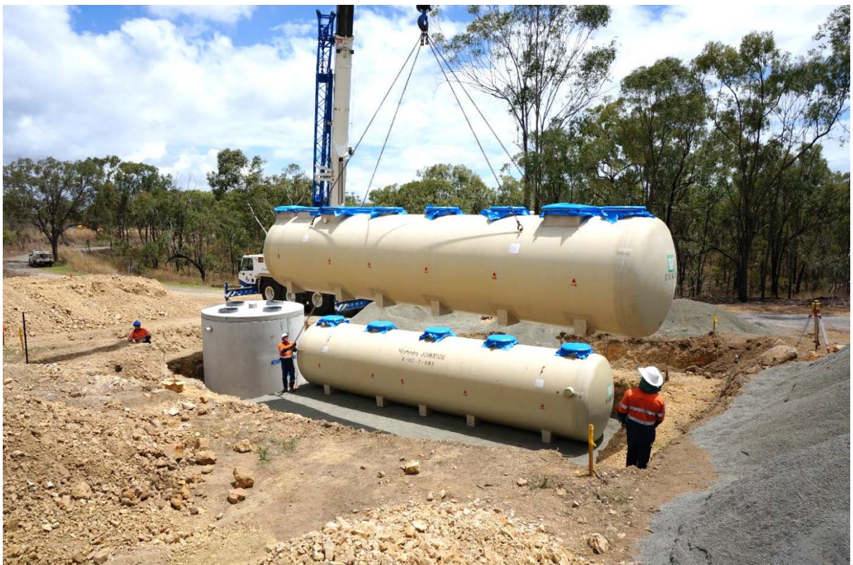
Figure 15 – The Kubota STP is lifted into place
